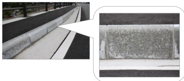
Figure 16 – Degraded GP walkway boundary block placed on strongly acidic soil (Beppu Myoban Spa, Oita, Japan)
